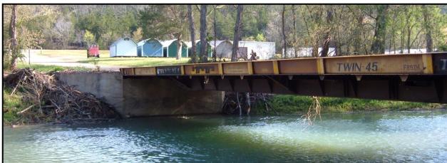
Bridge allowing sufficient water flow & fish passage.
